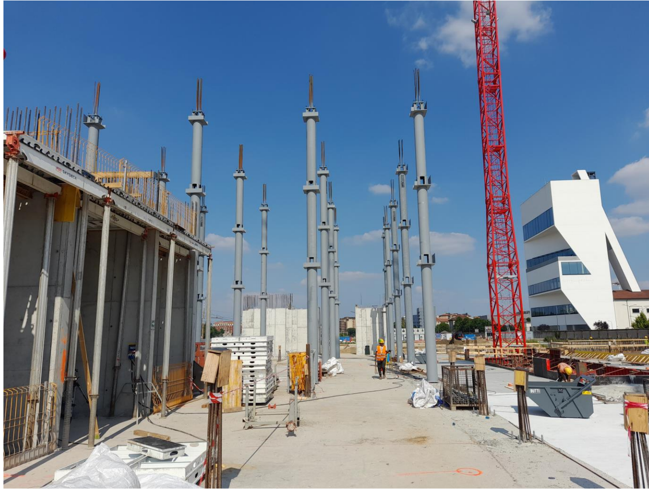
Prefabricated pillars - Building D
